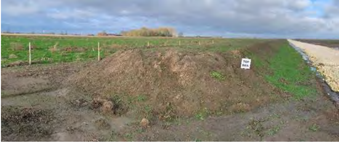
Insert 48: Topsoil storage for Viking Link Cable Works
