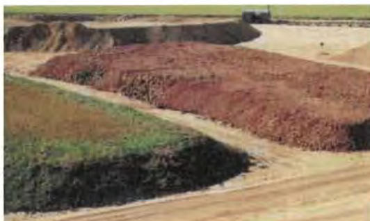
Clearly defined stockpiling of different soil materials
